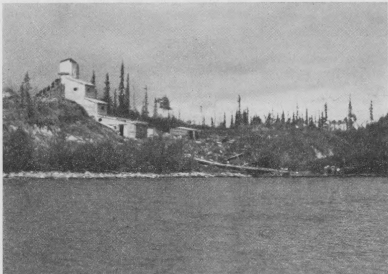
Pilot Mill on De Staffany Tantalum Beryllium Mines Limited Property at Great Slave Lake where beryllium, tantalum and columbium ores are treated
